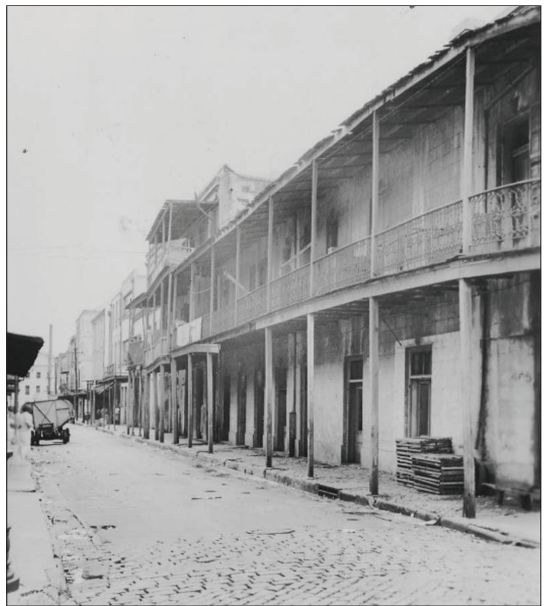
ABOVE: A view of the riverside buildings of Gallatin Street just prior to their destruction in 1935. The US Mint can be seen in the distance. Courtesy Louisiana State Museum. BELOW: An aerial view from 1922, courtesy Louisiana State Museum; annotation by Richard Campanella
